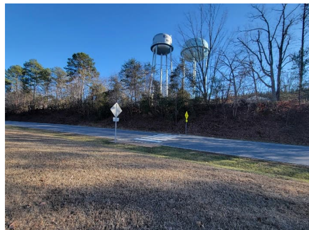
Crosswalks across US 70a at the CVS. Existing sidewalk is on the opposite side (south side) of the road heading west.
