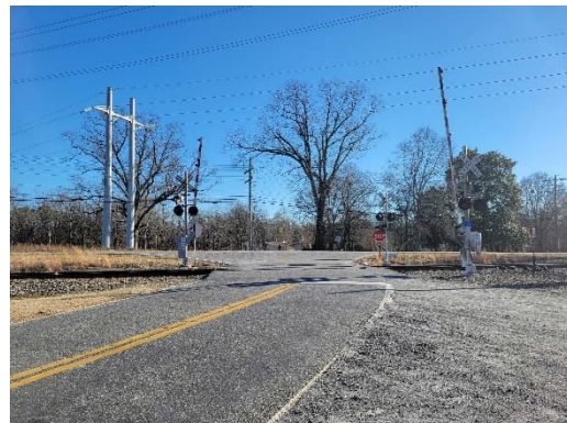
Tenth Street crossing of Norfolk Southern tracks (looking south)
